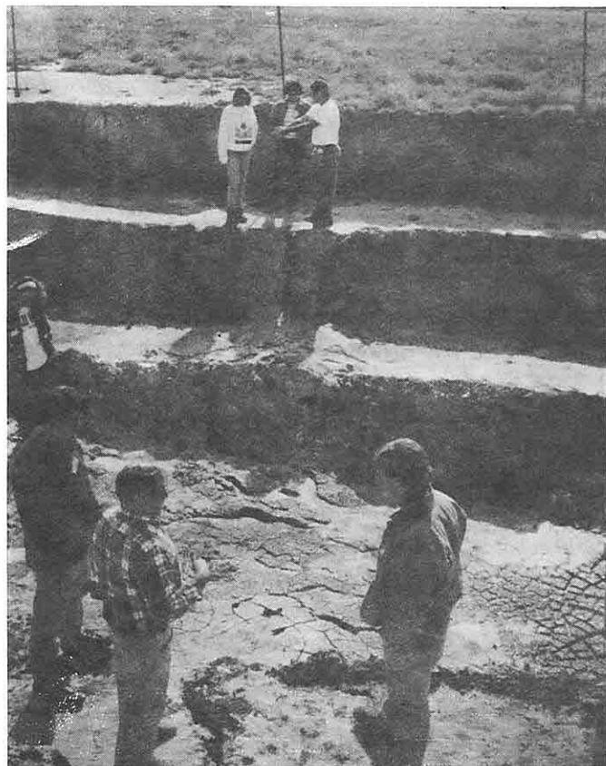
**Fig. 9.** Fissures exposed in a trench dug near the proposed site.
