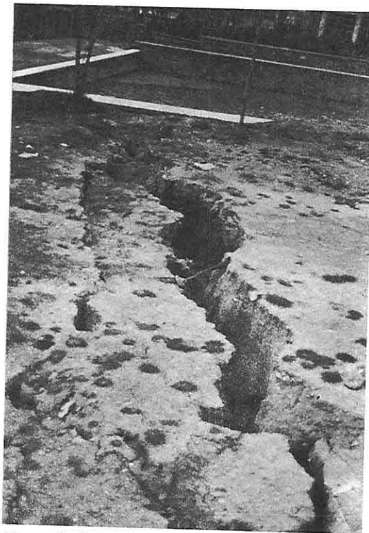
Figure 9. Large cracks extending across car park.
