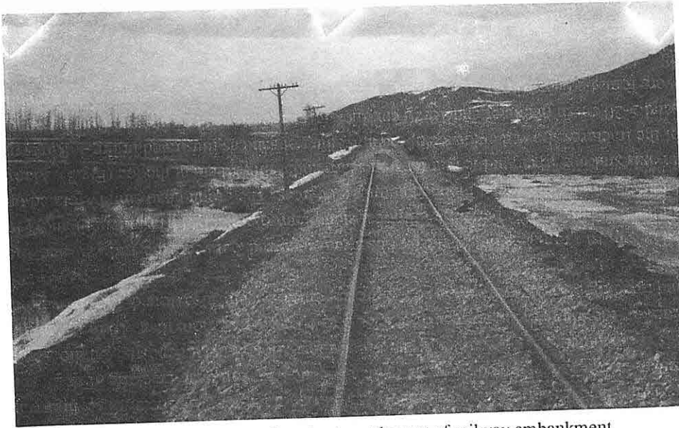
Figure 6. Railway bending due to settlement of railway embankment.
